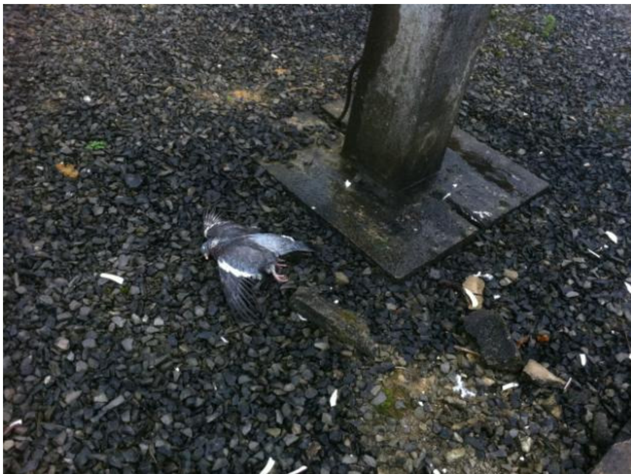
Photograph 1 – The dead pigeon and porcelain fragments at the foot of the support carrying the reserve 33kV bus-bar
