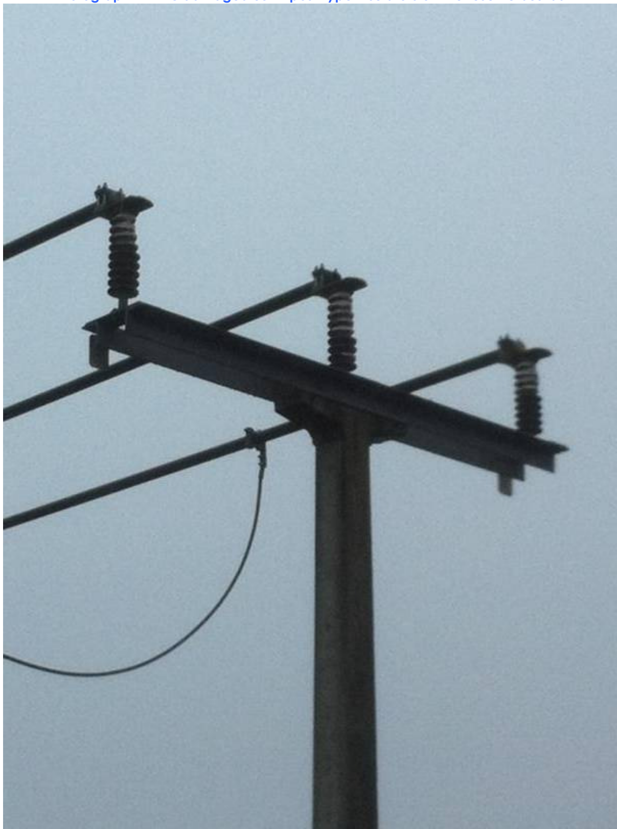
Photograph 2 – The damaged 33kV post-type insulators on the reserve bus-bar
